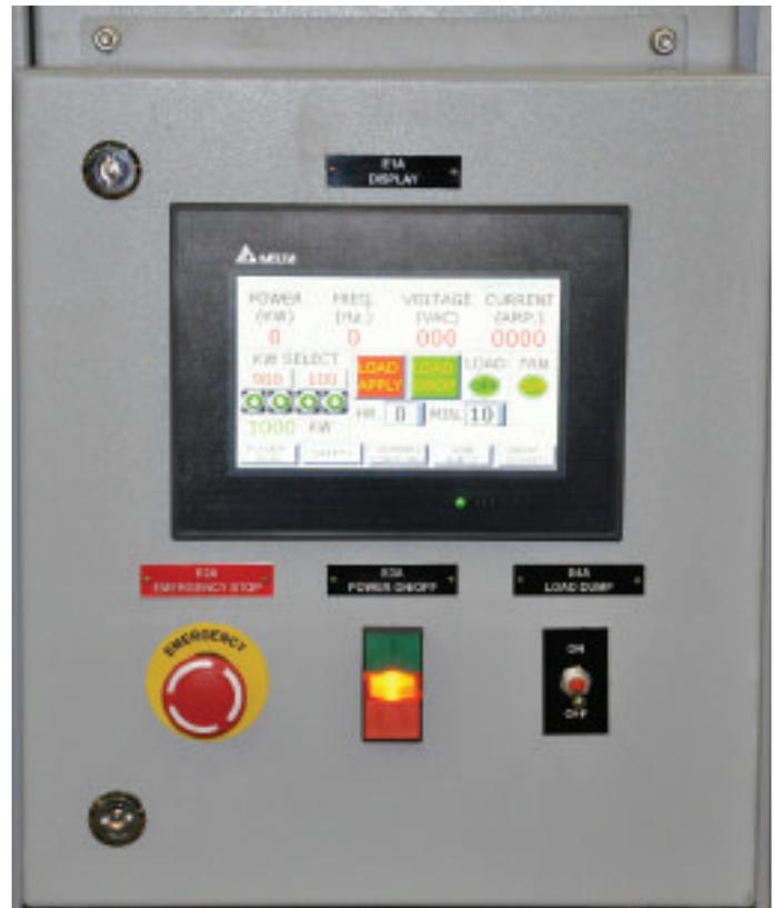
The TLB-R1000 load bank is digitally controlled via an onboard PLC with color touchscreen display. The control system includes standard data monitoring, such as voltage, current, kW and frequency, with test data able to be captured to a USB drive.
